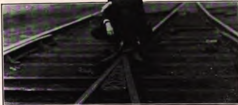
PLATE 17.—GUARD FOR FROGS MADE OF STEEL PLATE
